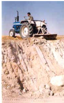
REMOVAL OF TOP SOIL
