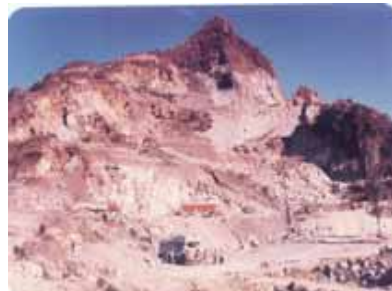
Overview during active mining (Limestone mine of MS. JST)
