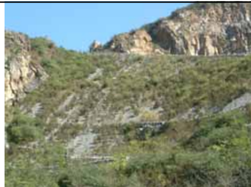
Dump Showing growth in greenery and stabalation after 2 nd rainy season
