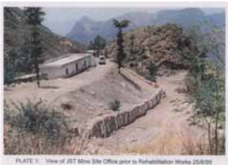
PLATE 1: View of JST Mine Site Office prior to Rehabilitation Works 25/6/99
