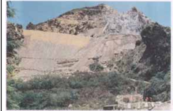
PLATE 3: View of JST Mine Dump after placement of Jute material and while right-hand side of Dump was being regraded
