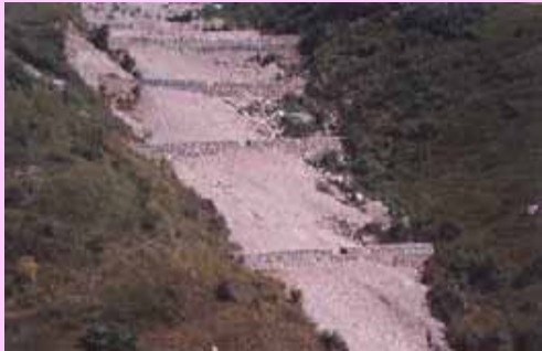
SHOWING A SERIES OF CHECK DAMS RAISED BY SH CHUHI RAM SHARMA BELOW THE MINE OF M/S SATYA TOMAR
