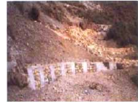
Showing Retaining Structure to retain debris
