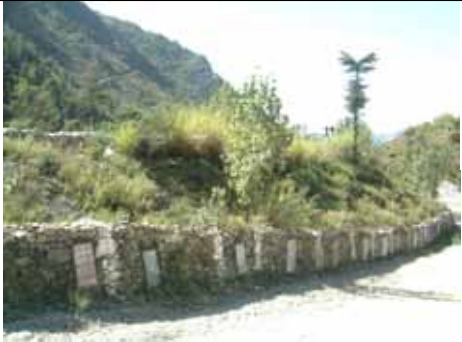
View of site after Rehabilitation
