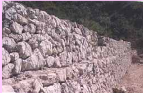
CLOSE VIEW OF CRATE-WIRE CHECK DAM
