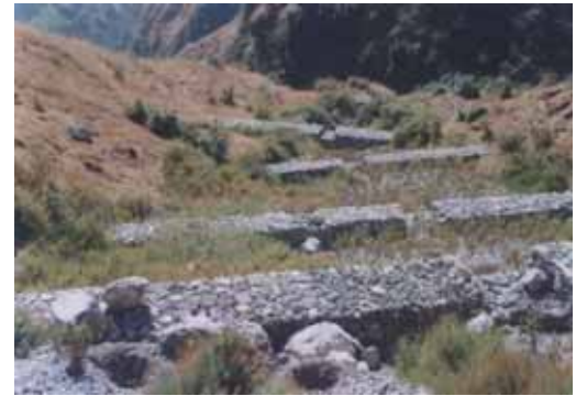
Plantation of Bushes in between check dams
